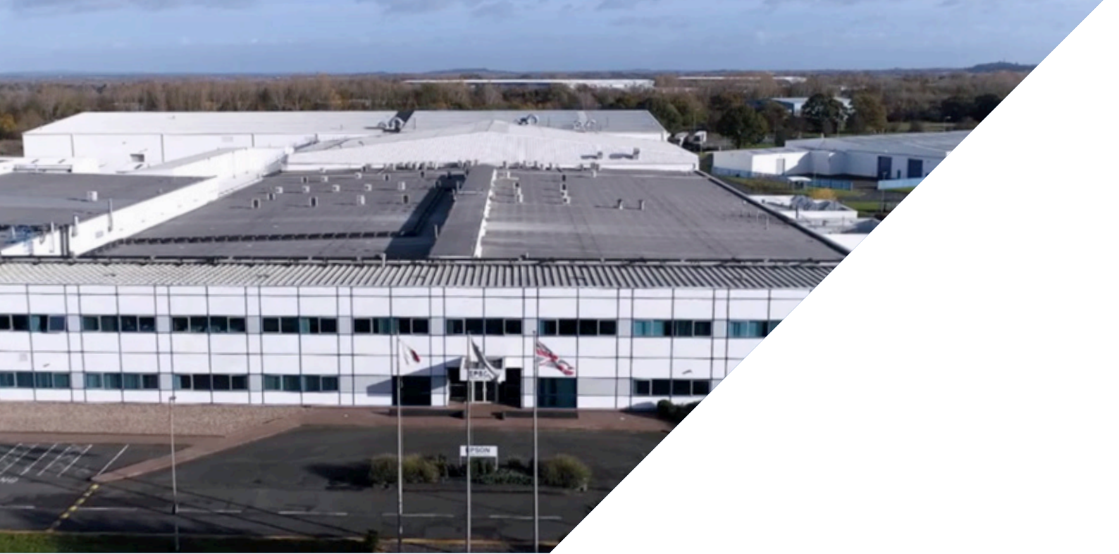
European manufacturing and distribution site, Epson Telford
